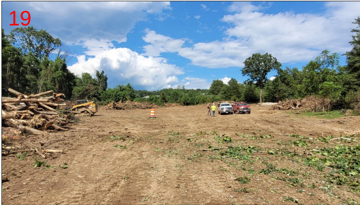
Site clearing and grubbing progress
