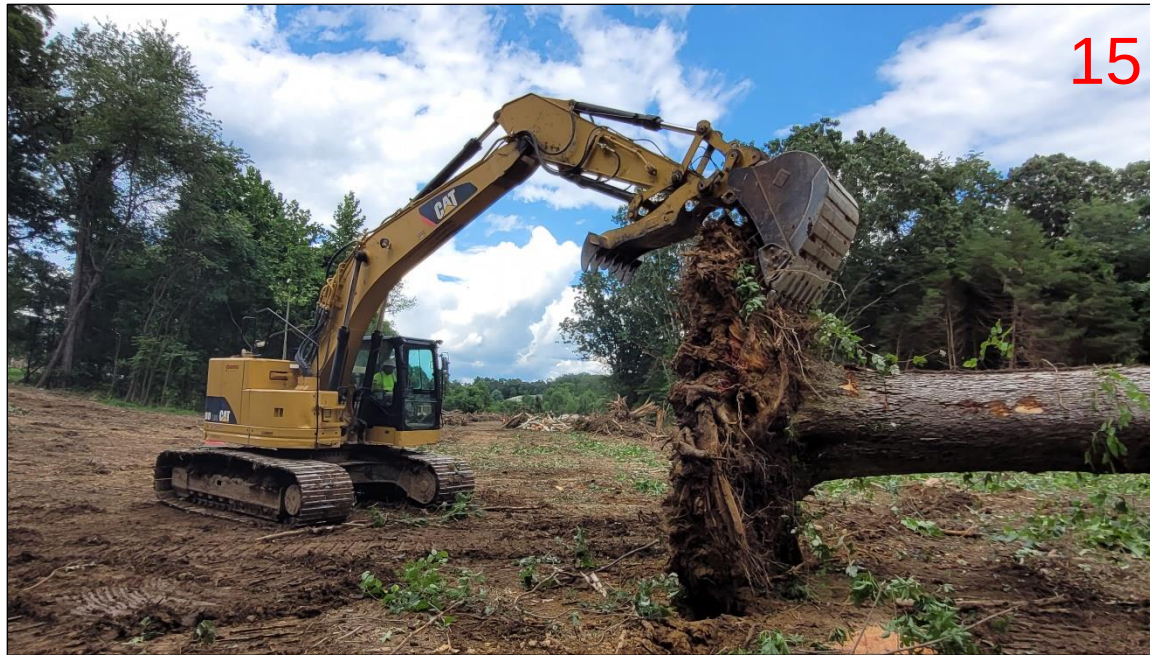
Site clearing and grubbing progress
