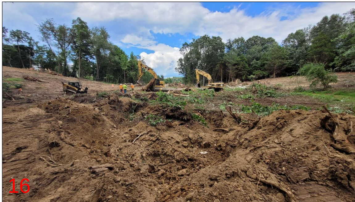
Site clearing and grubbing progress
