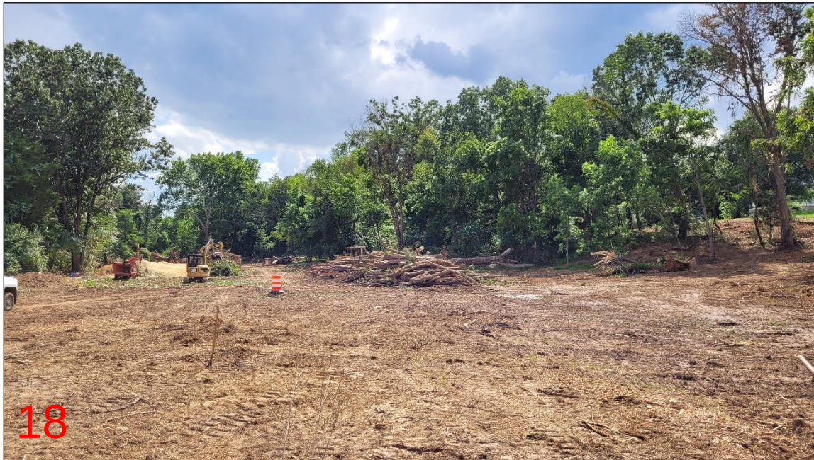
Site clearing and grubbing progress
